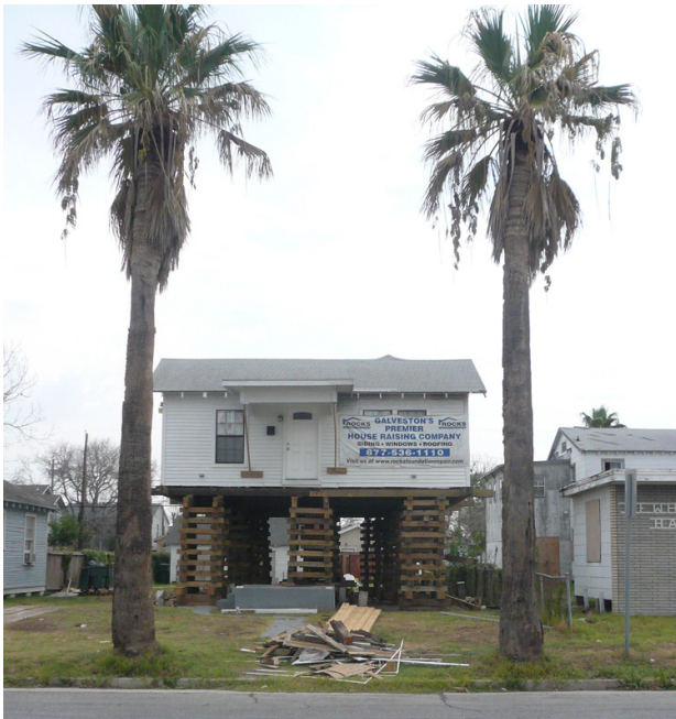
Figure 5. Previously flooded home raised to new BFE in Galveston.
